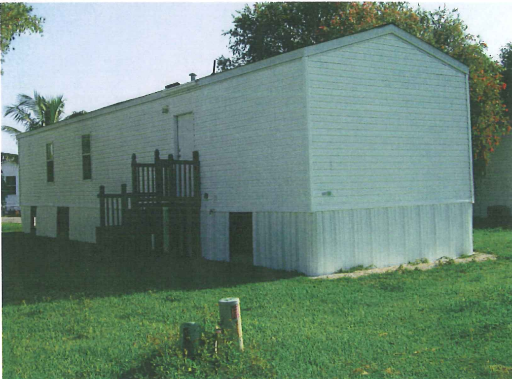
04/29/2016 West and south views
